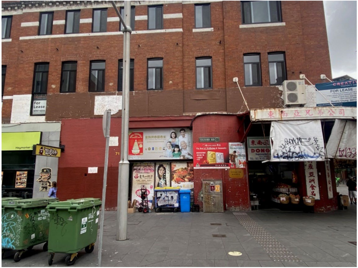
Ultimo Road looking south
